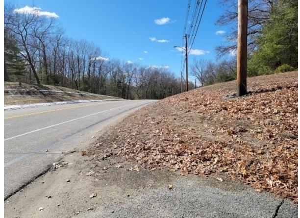
Looking to the west out of the proposed Barnum Road site driveway, the area is also sloped and grassed only. The tree line to the west is closer to Barnum Road. The photograph to the right shows the view measured 14.5 from the edge of travelled way. While it is the end of winter, the leaves from the previous Fall are still on the tree and do not block sight lines.
